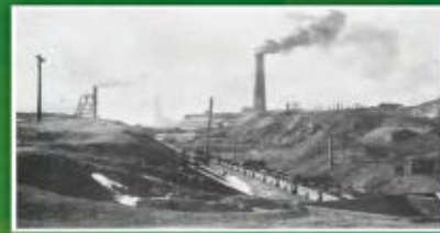
KOSAKA Mining was a leading Non-ferrous Mine in Japan.
