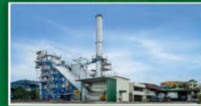
Vertical Stoker, an incinerator in Singapore, is first of its kind in South East Asia.
