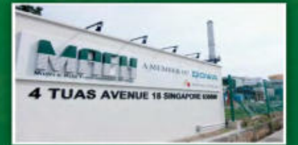
MAEH in 2019 - an amalgamation of Toxic Industrial Waste Treatment and Precious Metal Recycling Process.
