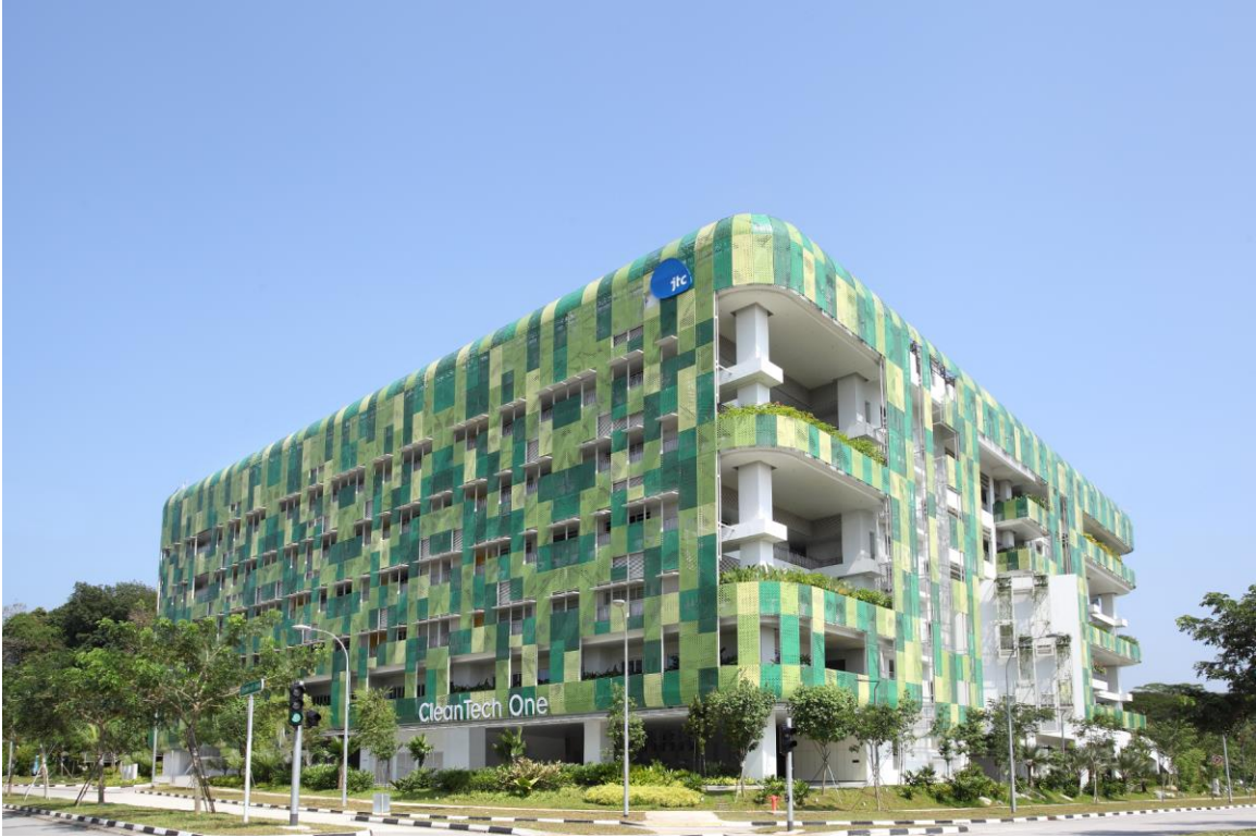
JTC CleanTech One @ Jurong Innovation District Credits: JTC
